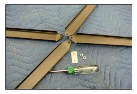
Place canopy connection bracket so that the PEM studs stick up through two brackets on the left, and two on the right. Use an 8-32 nut with captive star washer to secure brackets on stud (see below).
